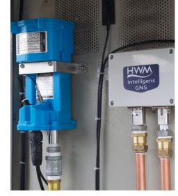
Intelligens is designed for use at pressure reduction points across the network, ensuring that pressures are within the specified range, without ever compromising a reliable supply.
